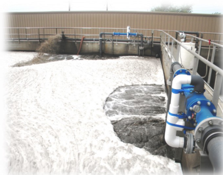
Aeration tank—Replacing diffusers
