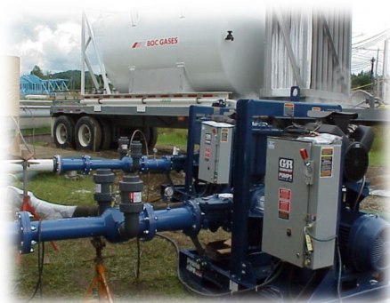
O 2 Injection—Replaces 2700 hp with 150 hp
