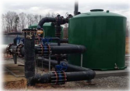
*Cylindrical Vessels:* made from heavy duty epoxy coated carbon steel or stainless steel and can handle flow rates up to 5000 CFM and 40 psig.
