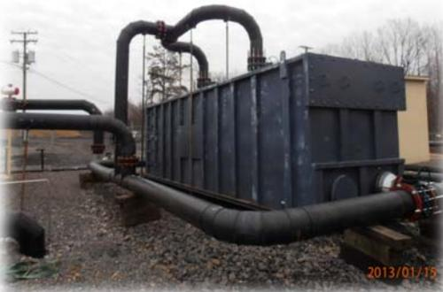
*High Flow Single & Dual Bed Vessels:* Box style vessels that can treat up to 10,000 CFM of gas in a single vessel.
