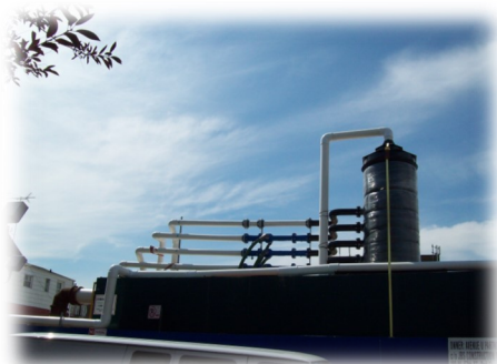
Stripping of VOC's & Gasses; Direct Oxidation of Iron & H 2 S without using Chemicals
