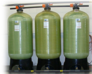
Mechanical Filtration for Removal of Suspended Solids, Metals, etc,
