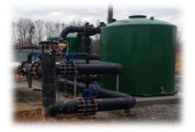
Cylindrical Vessels: made from heavy duty epoxy coated carbon steel or stainless steel and can handle flow rates up to 5000 CFM and 40 psig.
