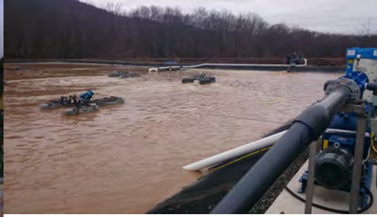
Aerating a wastewater lagoon - replacing surface aerators
