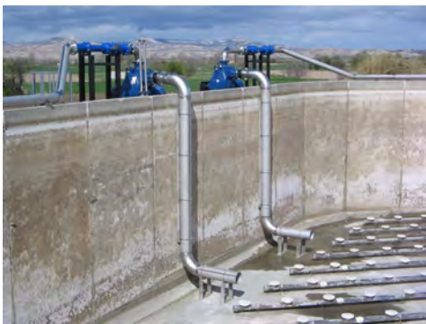
O 2 Injection—Replaces 1000 hp and hundreds of diffusers with 150 hp and two packages
