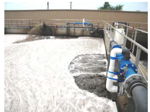
Aeration tank—Replacing diffusers
